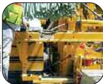
Trailing form with air-powered bar insertion.
