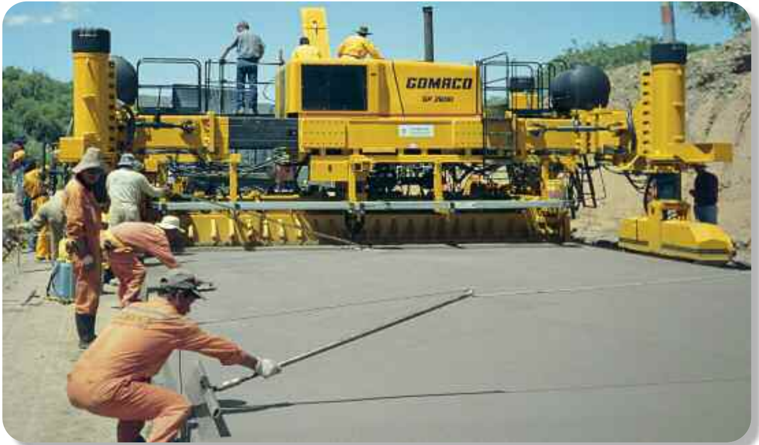
This versatile four-track GP-2600 slipforms a 24 feet (7.32 m) wide concrete roadway near Cochabamba, Bolivia.
