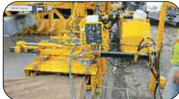
Female keyway with hydraulic side bar insertion (SBI) and vibration to the bar.
