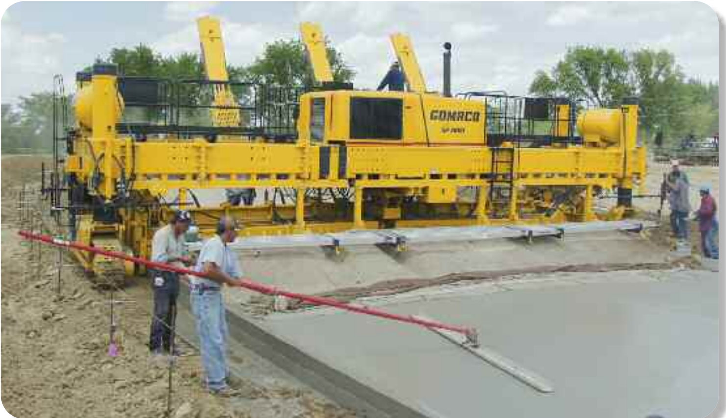
The two-track GP-2600 is slipforming a cul-de-sac with a 95 foot (29 m) inside radius. This machine is equipped with three frame-mounted bar inserters. This street in Wayne, NE, is being slipformed full width with integral curb on both sides.
