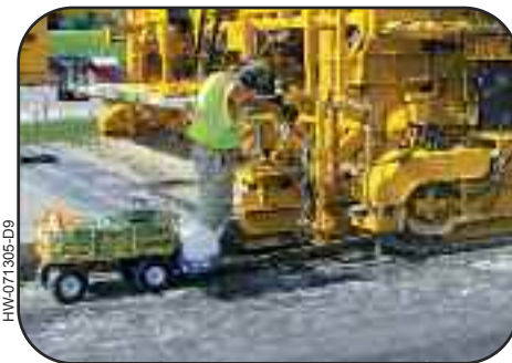
GOMACO's sideplate extension with the hydraulic system bar inserter.
