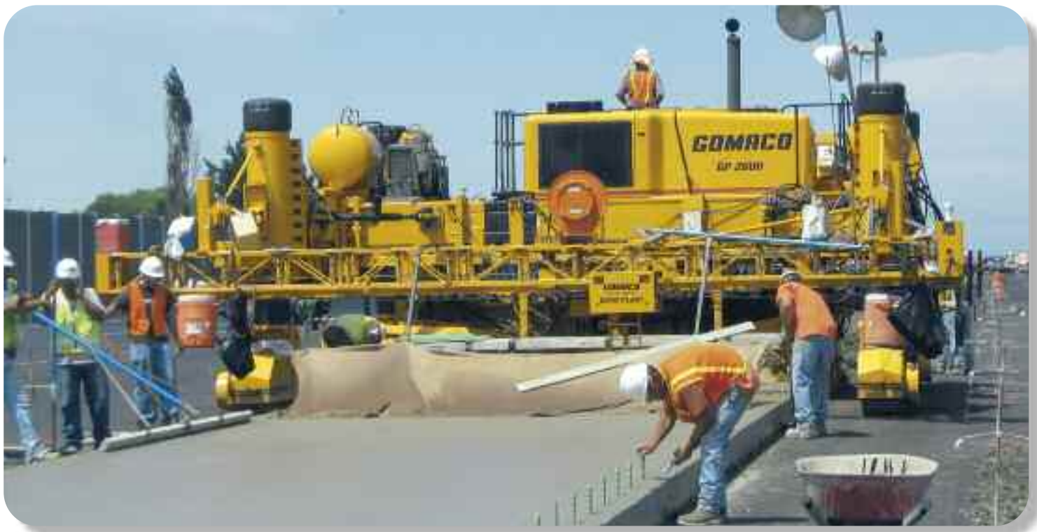
This versatile four-track GP-2600, equipped with the GOMACO Auto-Float®, slipforms mainline paving in Salt Lake City, UT.
