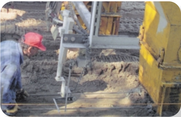
Specifications on this project in Kalamazoo, Michigan, called for steel being fed into the curb and gutter with the versatile GT-3600.
