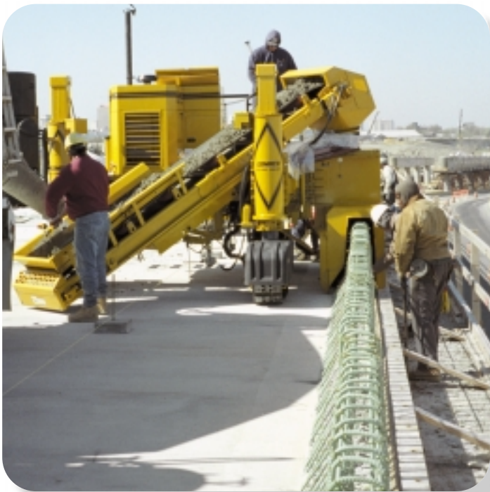
On this project, the GT-3600 slipforms 32 in. (813 mm) high bridge parapet over caged steel.
