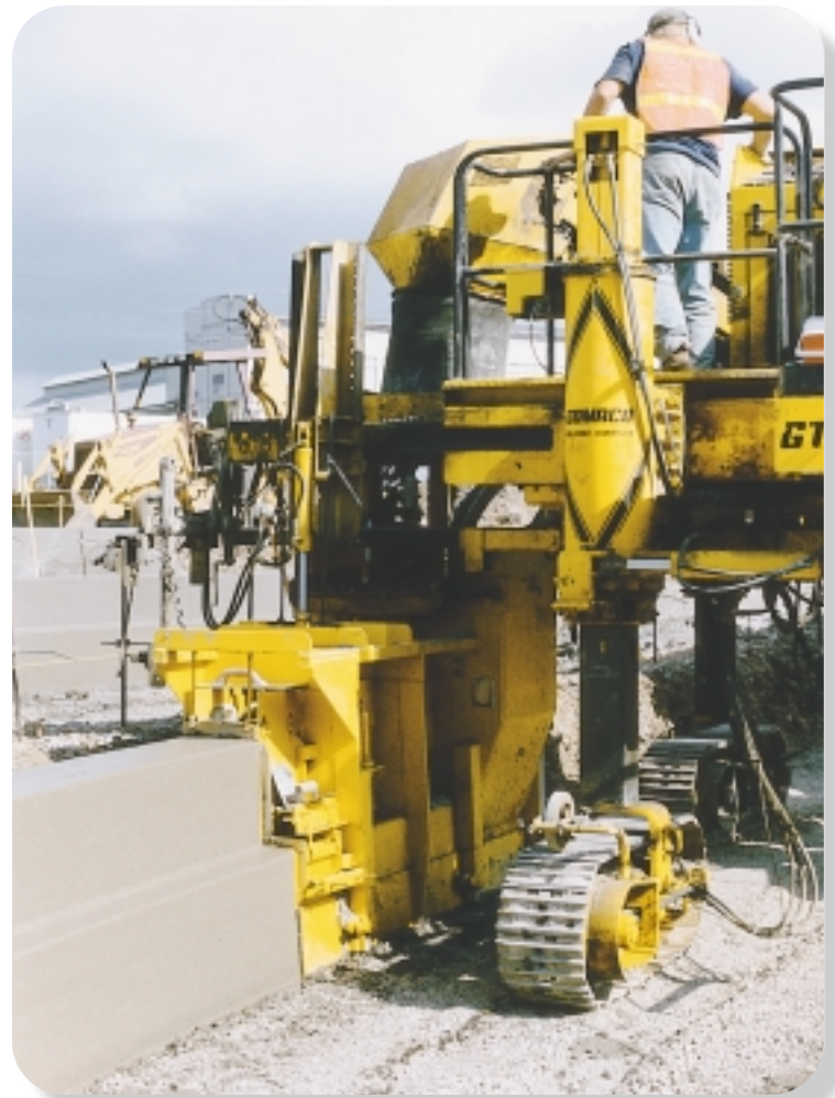
Another unique project involved the terracing for an amphitheater in Salem, Oregon. Retaining walls were slipformed with the GT-3600 at 34 in. (864 mm) high, with a 6 in. (152 mm) wide gutter/mowstrip, which was level with the backfilled grade.
