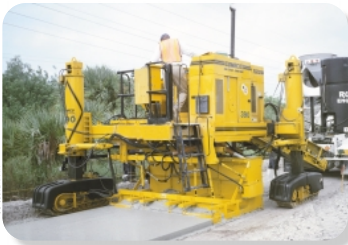
The GT-3600 slipforms 8 ft. (2.44 m) sidewalk on this residential project in Illinois.
