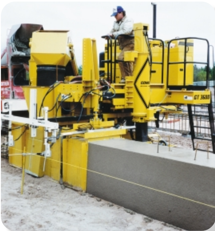
Another unique paving application slipformed with the GT-3600 is this foundation for an Ice Skating Rink.
