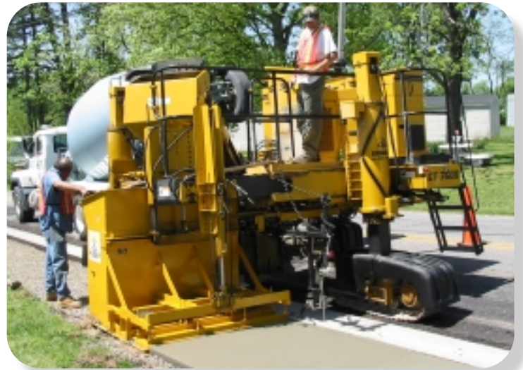
The GT-3600 (above photo) with All-Track Positioning (ATP) provides easy set up for slipforming sidewalk or (below photo) curb and gutter to the existing slab. Steering and grade is referenced off the existing curb or can be referenced off the stringline.
