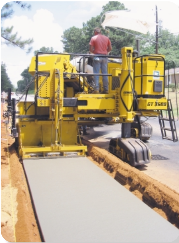
Minimum-clearance versatility, and high production is achieved with the GT-3600, slipforming this 5 ft. (1.52 m) sidewalk in Alabama.
