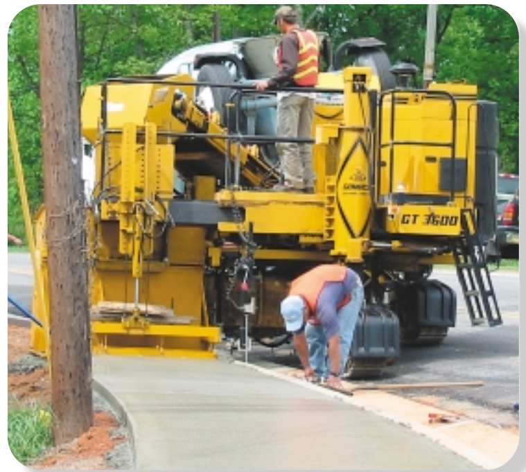
Minimum clearance on the GT-3600 provides the ability to avoid obstacles such as telephone and light poles. Steering and grade is referenced off the existing curb on this scab-on sidewalk project.
