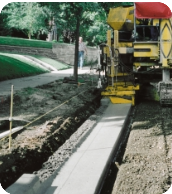
This GT-3600 has a Guillotine-style curb depressor.
