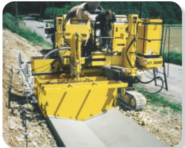
The versatile GOMACO GT-3600 slipforms drainage canal in France. The sidemounted design allows minimum-clearance on the left side of the mold.
