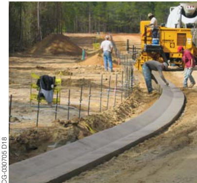
Roll-over curb is one of many profiles the GT-3200 can slipform.
