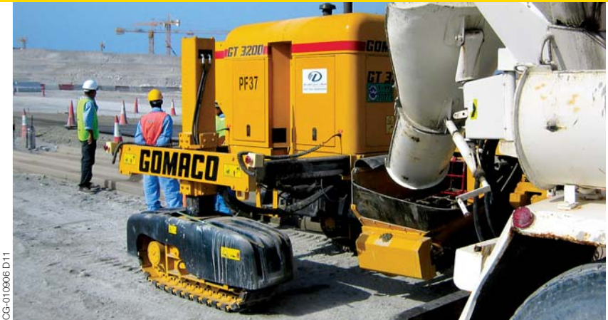
The GT-3200's powerful auger moves the concrete into the machine's hopper.
