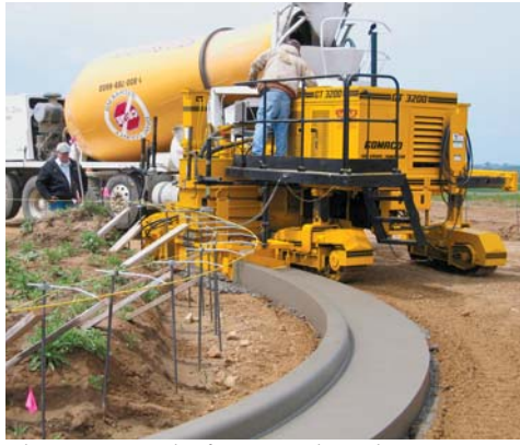
The GT-3200 slipforms curb and gutter around a radius on a subdivision project.
