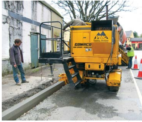
New stand-up curb is the first step for this street rehabilitation project.
