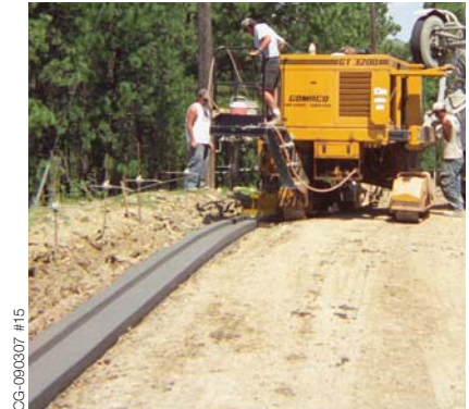
The GT-3200 slipforms channel footing in a historic cemetery.
