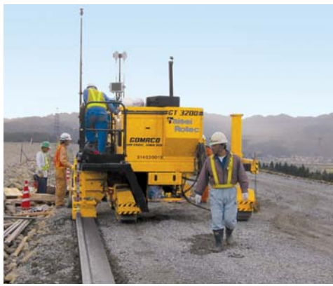
The GT-3200 can be controlled with stringless guidance systems.
