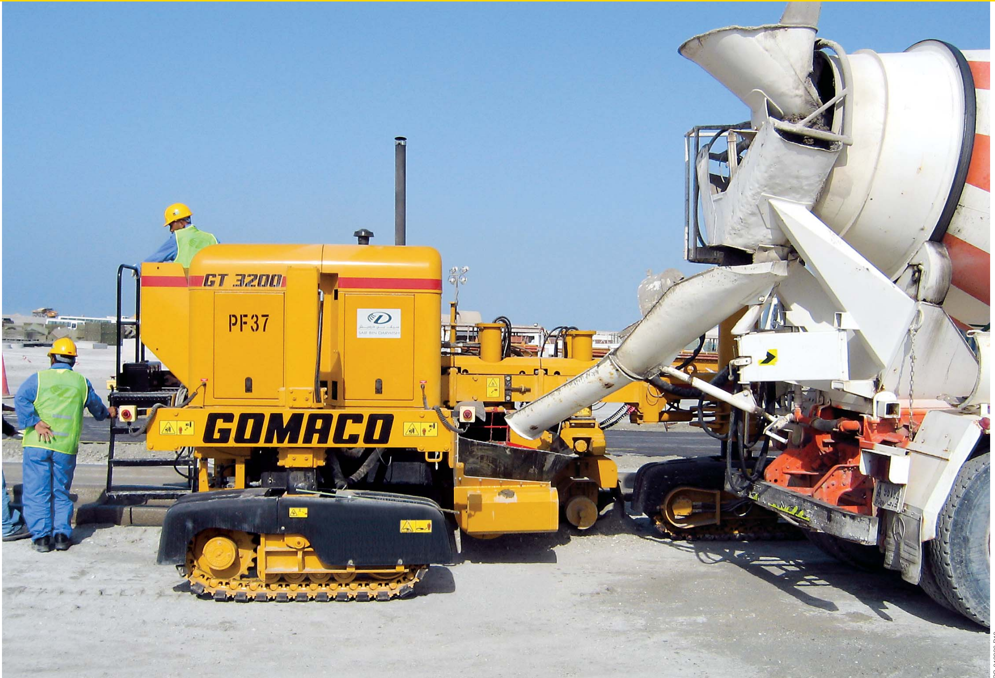
A GT-3200 with auger system slipforms curb and gutter on a project in Abu Dhabi, UAE.
