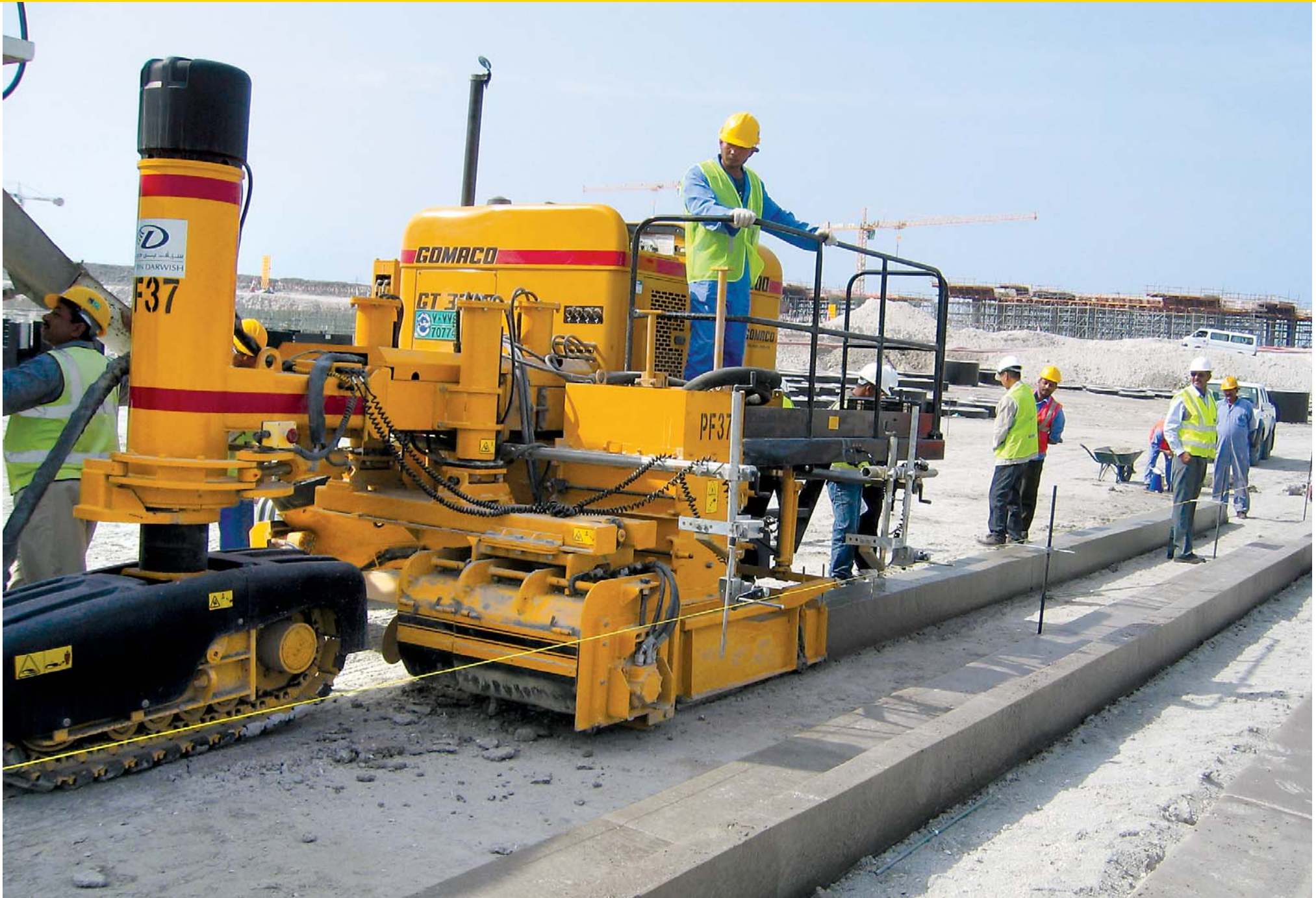
A contractor in Abu Dhabi, United Arab Emirates, conducts a test pour with their new GT-3200 to learn the operation of the machine and perfect their concrete mix design.
