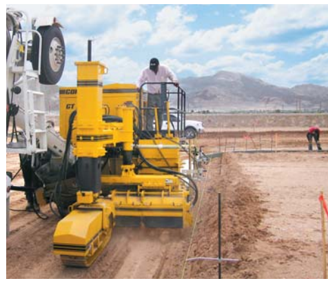
New curb and gutter goes around a radius for a brand new roadway project.
