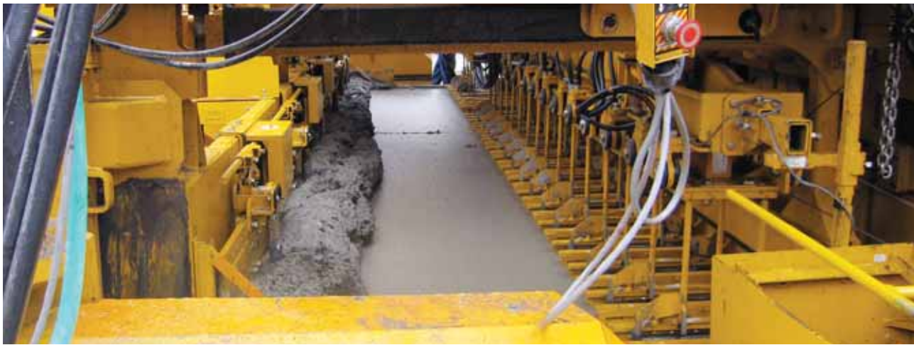
The IDBI attachment's finishing process includes a tamper bar, unique oscillating straightedge, paving pan and stainless steel that follow the bar inserters and repair scarring from the insertion process.
