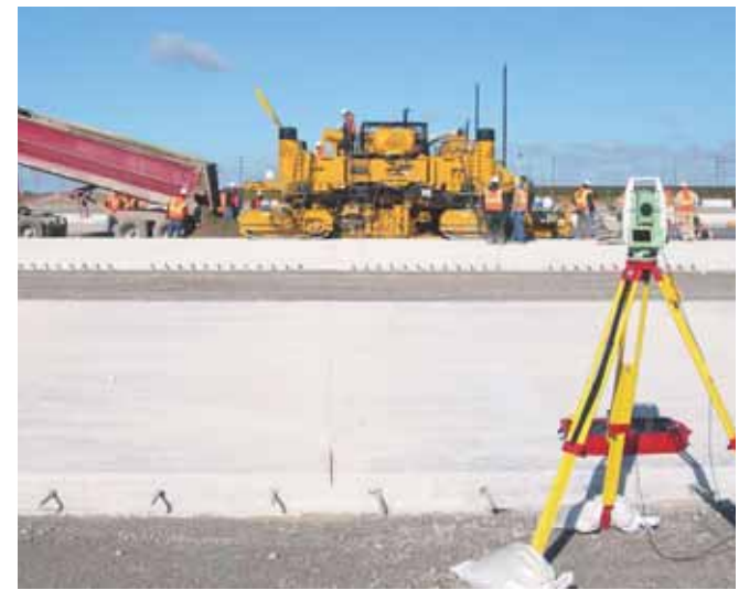
The GOMACO GHP-2800 with an independent IDBI attachment slipforms with a Leica stringless guidance system.
