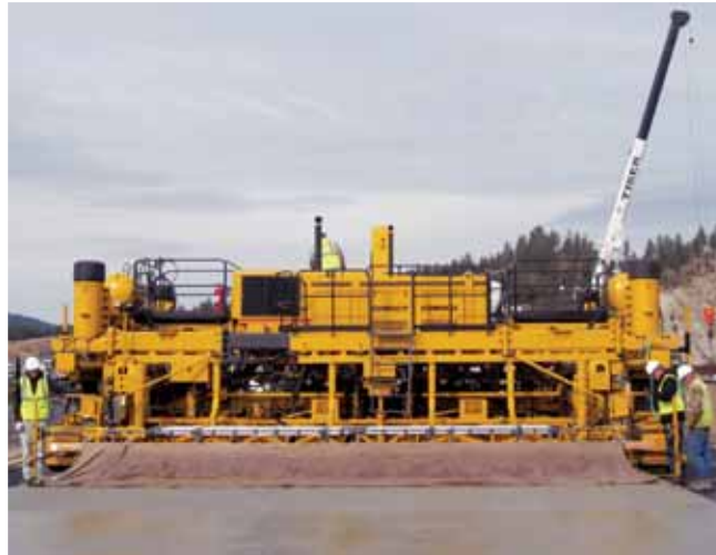
The independent IDBI attachment provides time and labor savings with on-the-go placement of dowel bars across the width of the slab.
