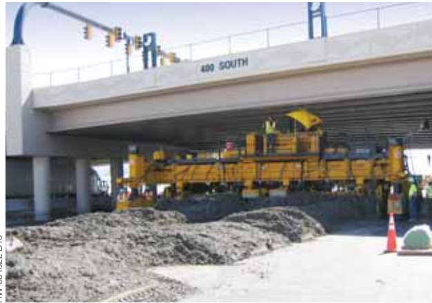
A GP-4000 with IDBI attachment has plenty of clearance as it slipforms underneath a bridge overpass.
