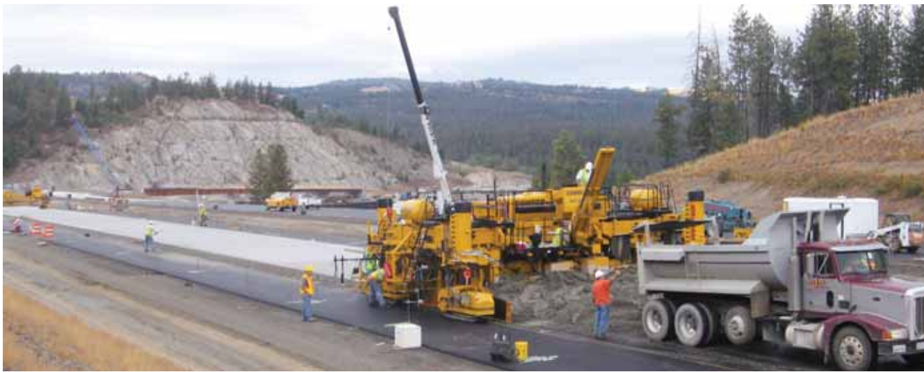
A CAN cable connects the controllers on both the paver and the IDBI allowing the two systems to communicate. For example, when the paver stops and starts, the tamper bar and screed on the IDBI turn on and off automatically coordinating with the paver.
