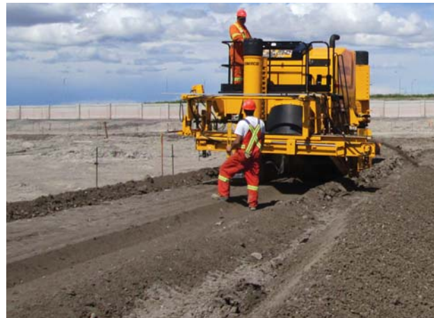
The transfer conveyor has seven feet (2.1 m) of sliding capabilities to place the material over the stringline or into the center of the road.
