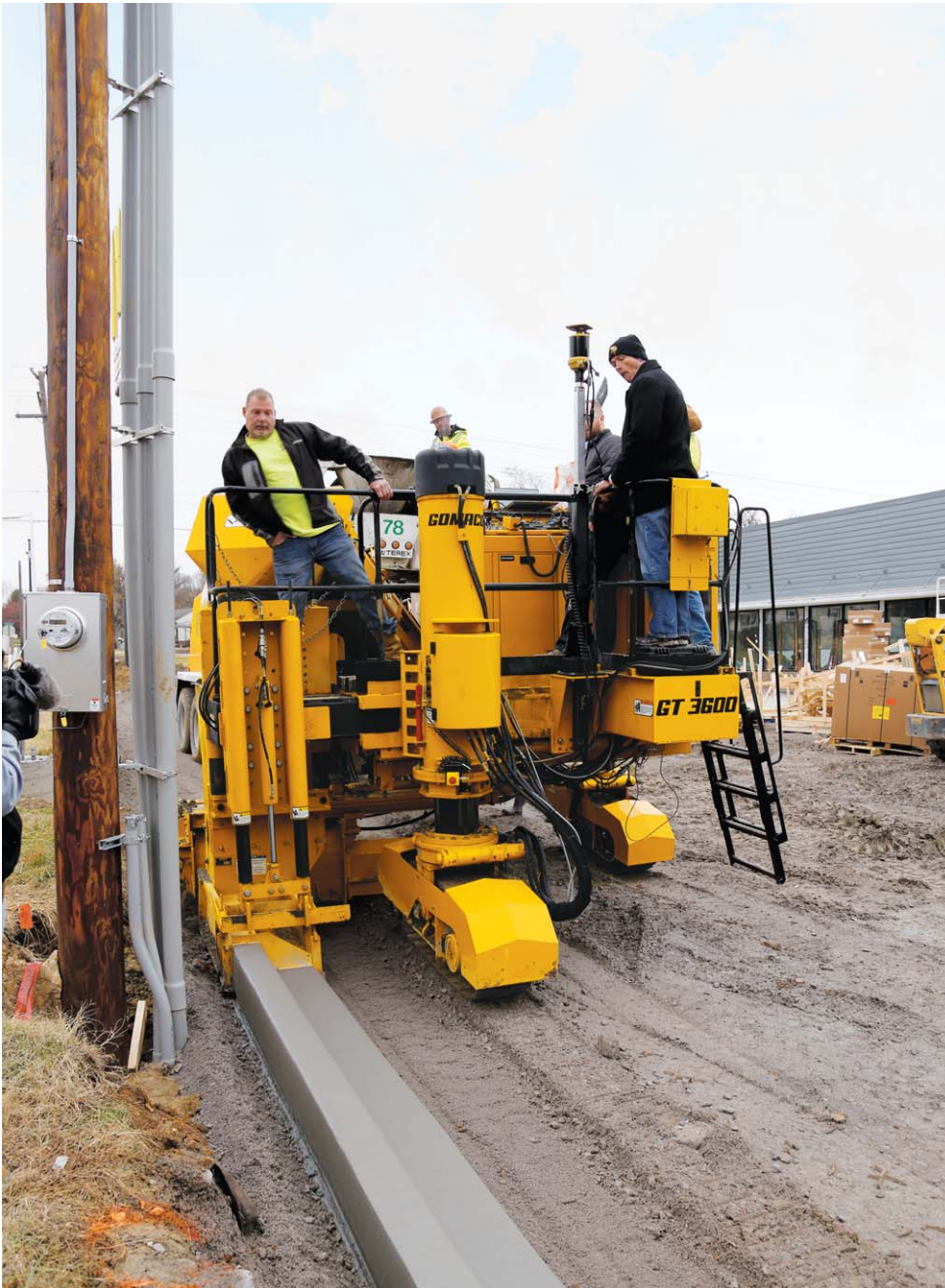
The Xtreme GT-3600 slipforms curb and gutter using 3D machine guidance to maximize the Xtreme GT-3600's minimum-clearance capabilities.
