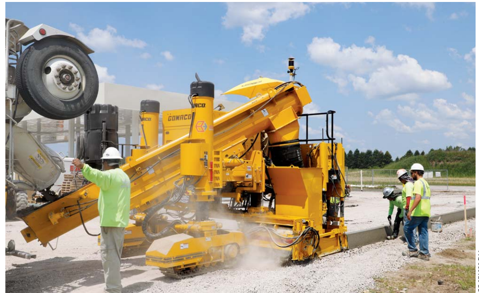
The ability to trim and pour curb and gutter in one pass is just one of the time and money saving capabilities with the Xtreme GT-3600. The trimmerhead is direct-driven with a radial piston hydraulic motor which provides maximum torque for trimming capacity.
