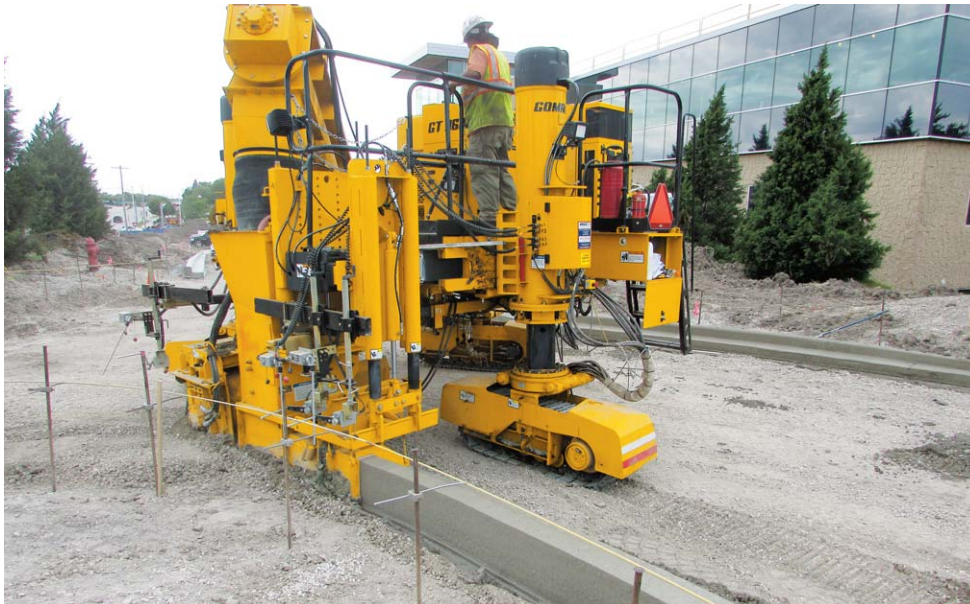
The Xtreme GT-3600 features the GOMACO three-sensor radius system for stringline. When paving with stringline, the lead steering wand is allowed to leave the stringline and reference is switched to sensor number two for traveling around the tight radius.
