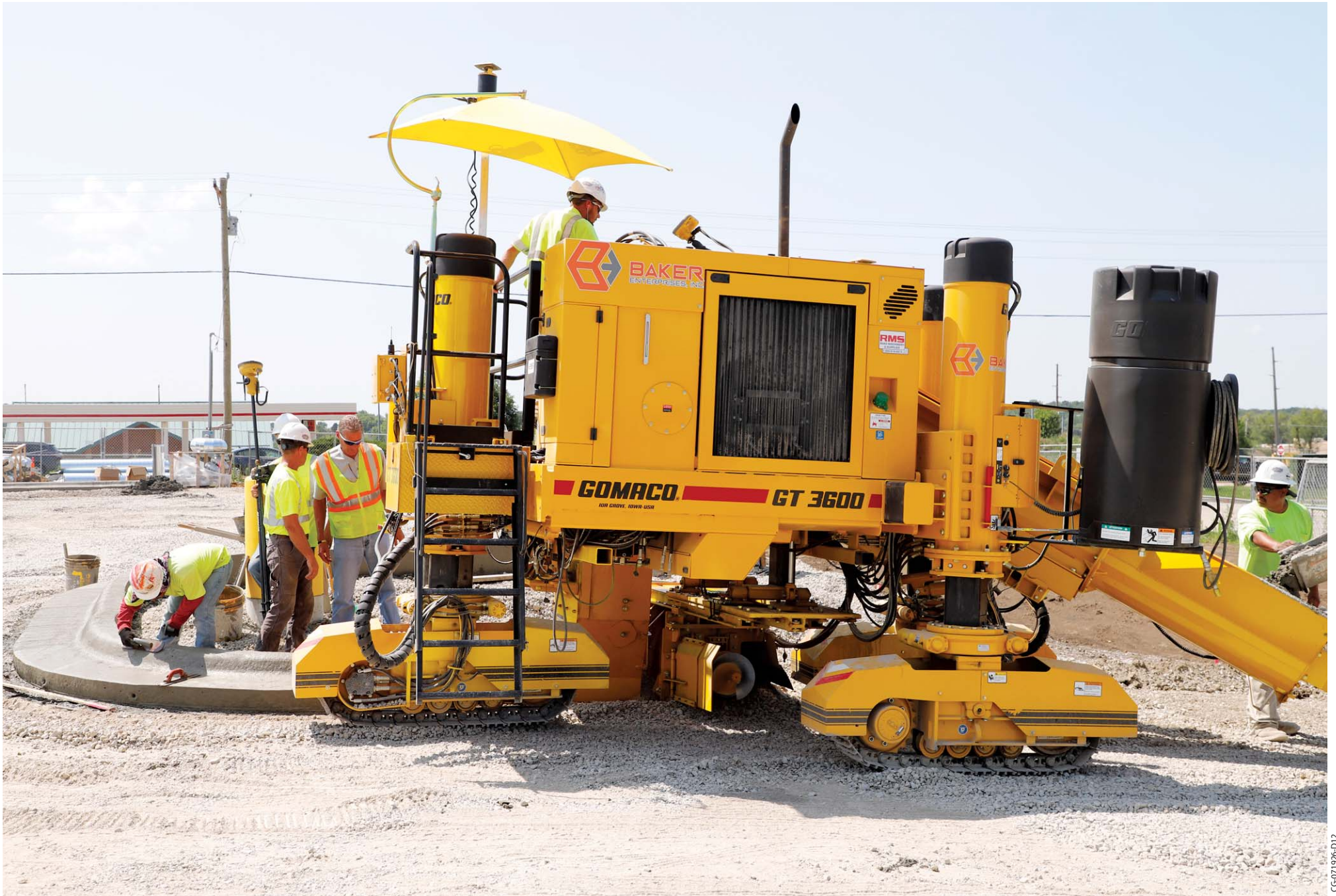
All the capabilities of the Xtreme GT-3600 allow you to quickly and efficiently pour today's parking lot designs for curb and gutter.
