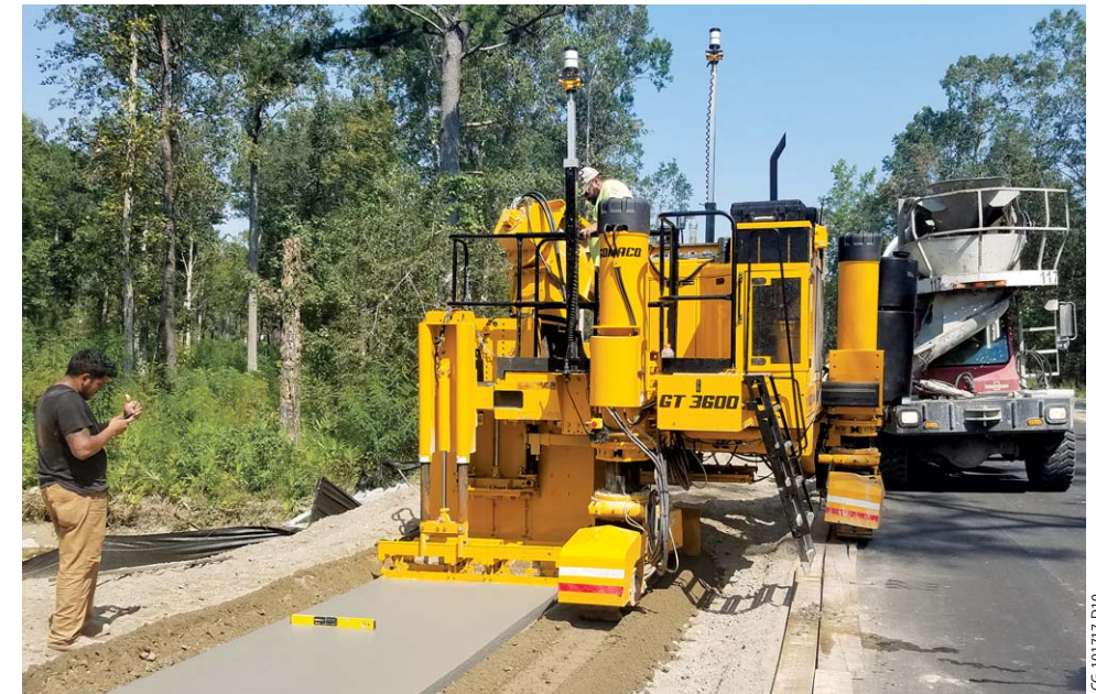
A GOMACO Xtreme GT-3600 slipforms a five foot (1.52 m) sidewalk with 3D machine guidance.
