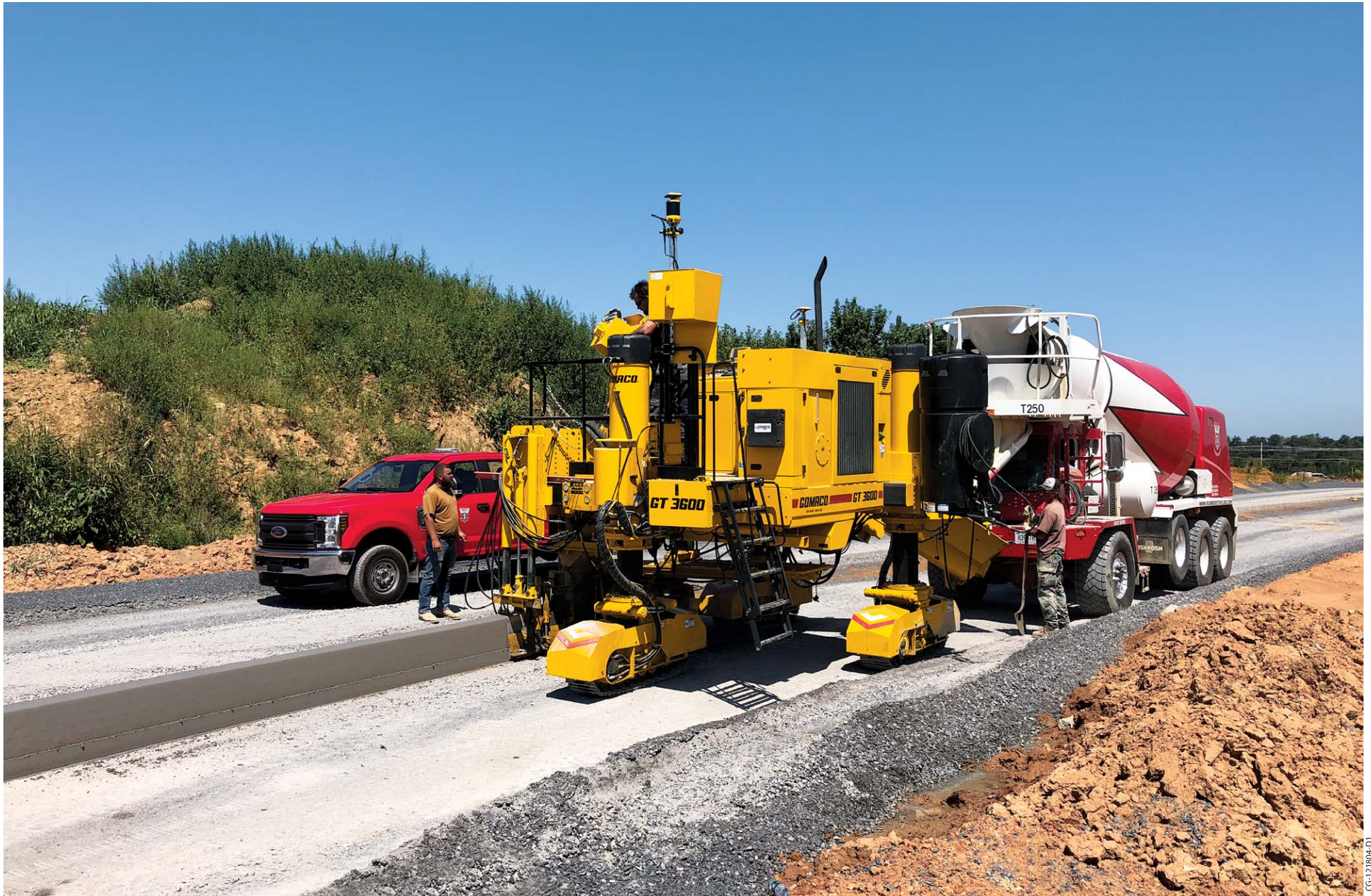
The GOMACO Xtreme GT-360 is slipforming an 18 inch (457 mm) stand-up curb and is equipped with the GOMACO Remote Diagnostics (GRD) allowing for remote upgrades and fleet management from a cell phone or laptop computer.
