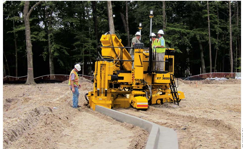
The intelligent All-Track Positioning on the Xtreme GT-3600 includes a smart hydraulic cylinder on all three legs. The smart cylinders allow G+® to know the position of all three tracks and can make steering adjustments as needed.
