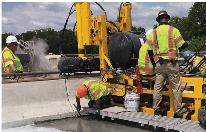
Zero-clearance UHPC paving can be accomplished with the ability to position the legs of the paver where they need to be.
